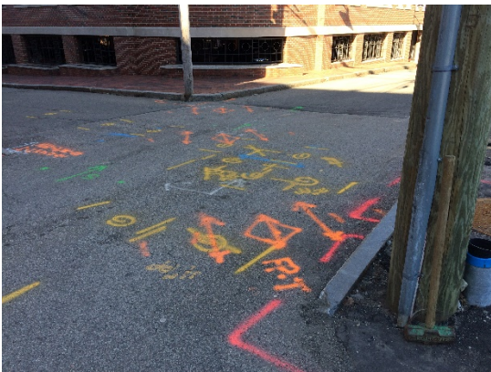
Multiple utility conflicts at Chestnut & Porter
